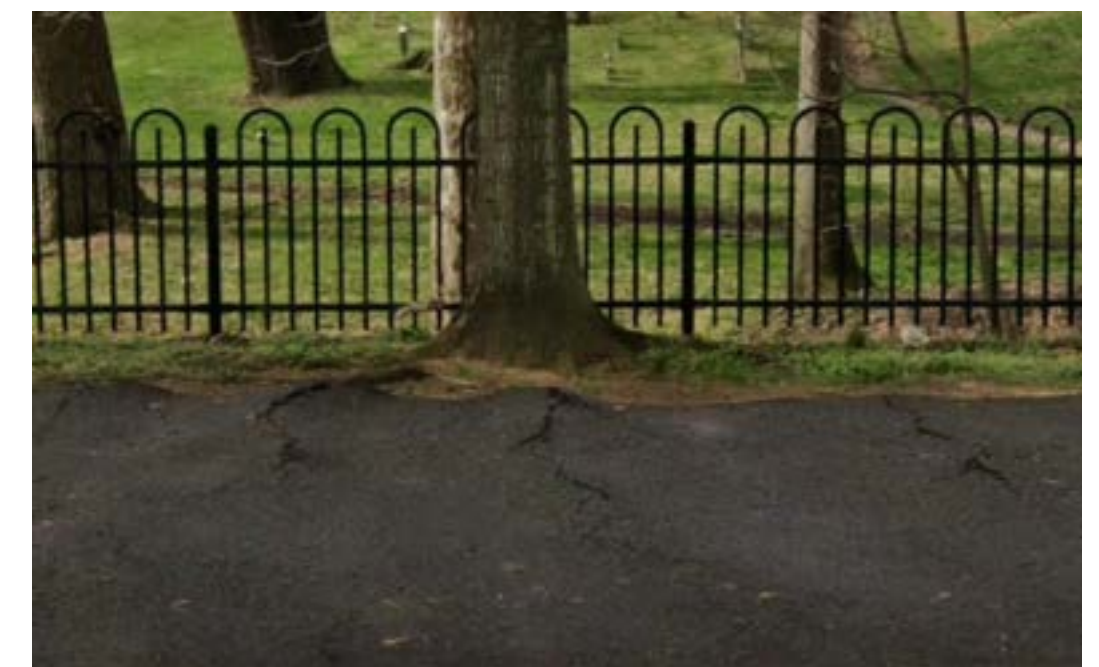
Tree root damage along Jamieson
